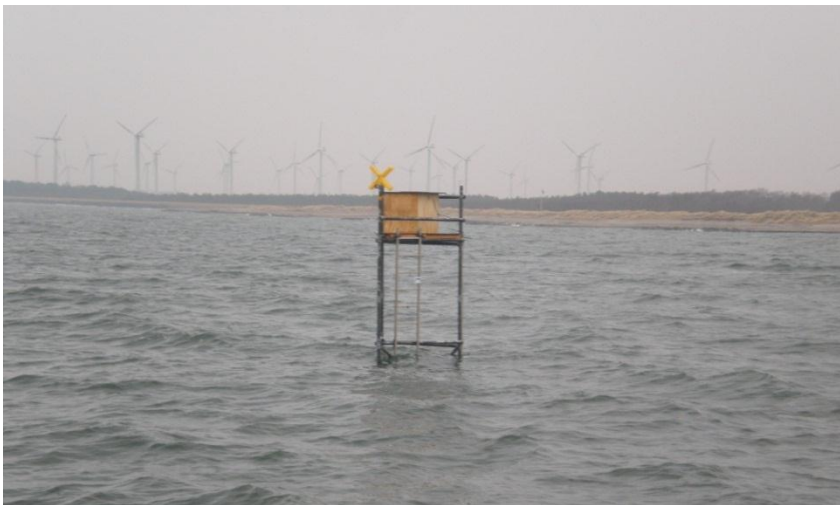
Figure 3.6 View of the automatic water sampling station at NS03a
