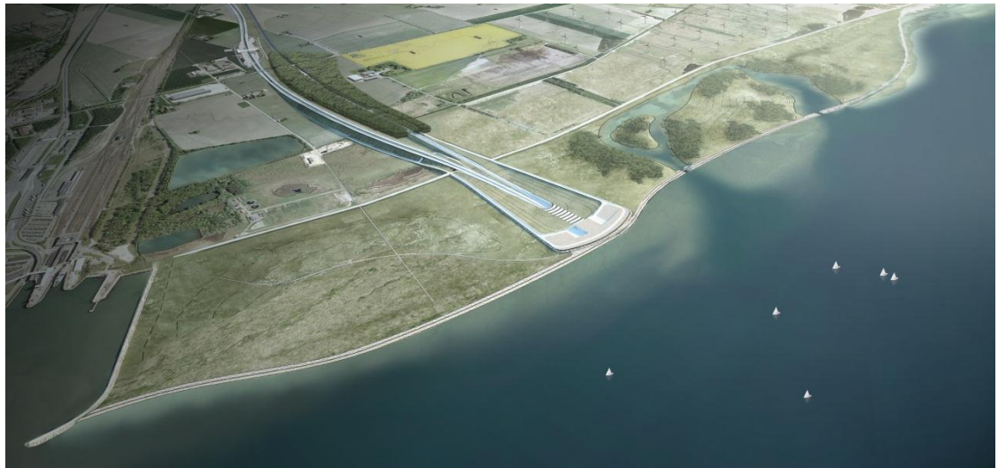
Fig. 2.5 Tunnel portal area at Lolland
