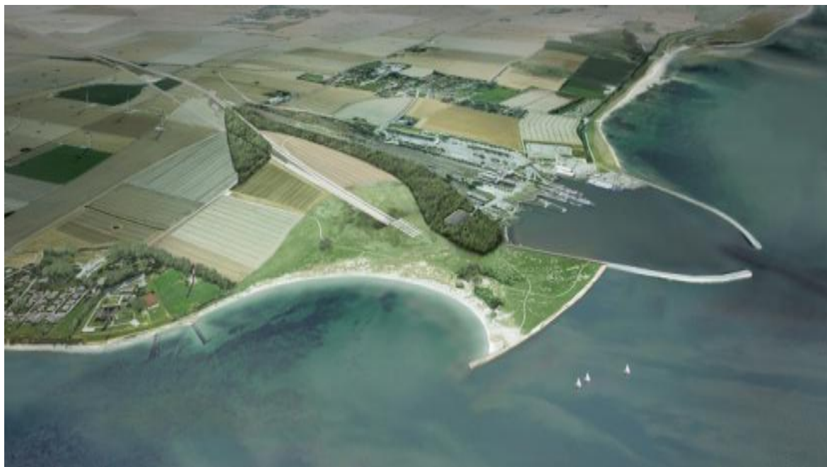
Fig. 2.4 Reclamation area at Fehmarn
