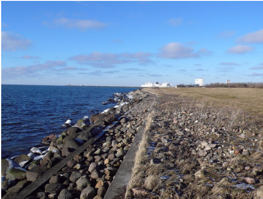
Figure 5.22 Existing revetment along the coast where the marine ramp and beaches are planned
